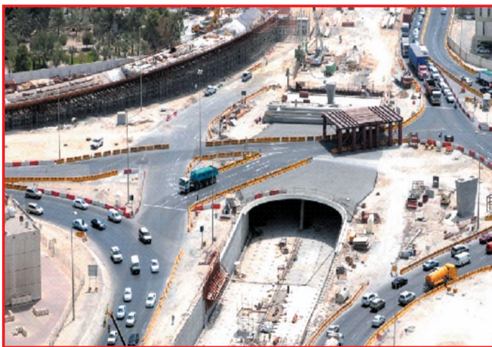
● Work on the Shaikh Isa bin Salman Highway underpass
